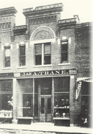
Trane Storefront La Crosse, Wisconsin 1891
